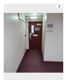
FULL ACCESS **Inspection Type Fire Door Condition** X The leaf and frame are adequately specified Replace door with FD30s rated fire door. **NO TIMESCALE** The door is not fit for purpose - 38mm hollow. REFERENCE RB-U96ZMD DUE No Due Date **NO SEVERITY**
