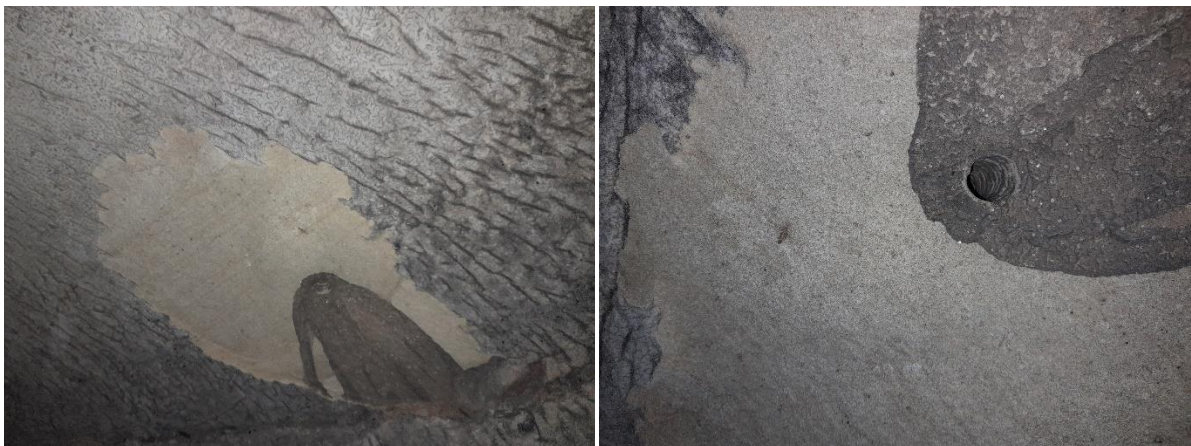
Impact of Cave Probing including localised area of spalling and later water ingress (Credit: Tim Allen)
