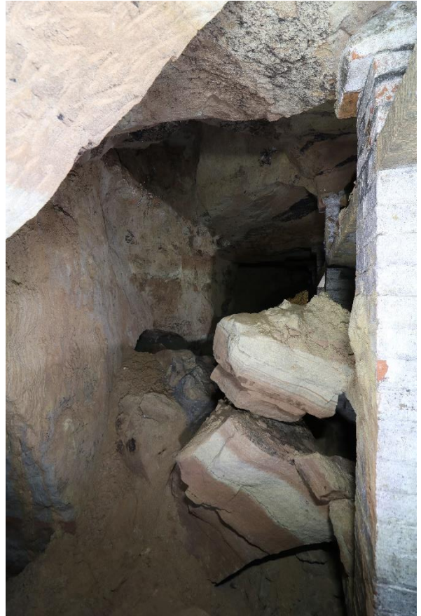
Partial collapse of the ceiling of a cave at Wollaton Hall due to water ingress
