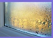
Condensation mainly occurs during the colder months, whether it is rainy or dry outside. It is usually found in the corners of rooms, north facing walls and on or near windows. It is also found in areas of poor air circulation such as behind wardrobes and beds, especially when they are pushed up
