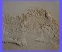
Rising damp will be present all year round but is more noticeable in winter. If left untreated it may cause wall plaster to crumble and paper to lift in the affected area. Note. Black mould will not usually be seen where there is rising damp. This is because rising dampness carries with it ground salts which prevent the growth of black mould. However secondary factors can result in conditions becoming varied.
