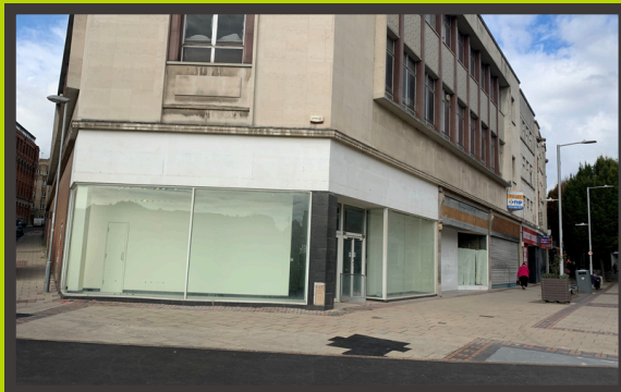
Lister Gate Art Project - before
