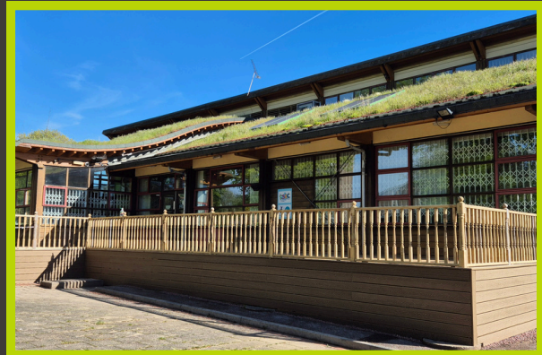
Decking at St Ann's Advice Centre - St Anns
